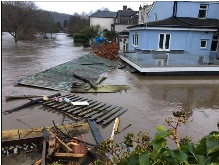
Figure 5: Image showing the overtopping of the River Taf to the rear of Cardiff Road which submerged the rear gardens and ground floor of several properties during Storm Dennis (image provided by resident)
