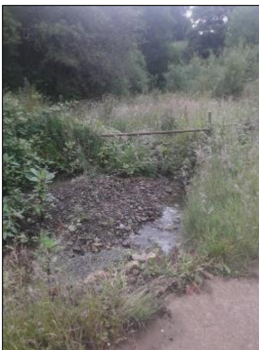
Figure 20: Image of debris accumulation within the unnamed ordinary watercourse channel upstream of 'Culvert Inlet 1' (Figure 4) (captured during CCTV operations on 30/06/2020)
