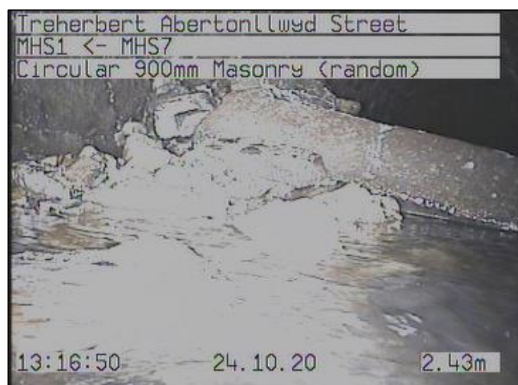
Figure 15: Internal view of 'Abertonllwyd Street Culvert Network 1' downstream of 'Manhole 1' (CCTV survey footage captured 24/10/2020)
