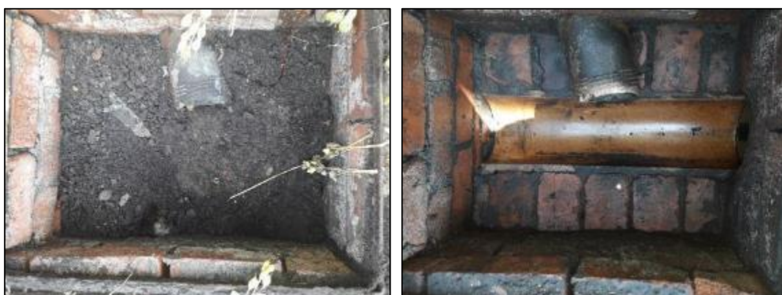
Figure 15: Photo of a manhole at Oxford Street captured before (left) and after (right) surveying and cleansing operations during June 2020
