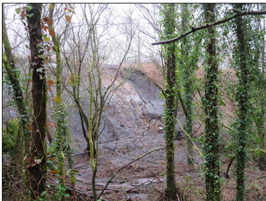
Figure 4: Landslip of the hillside above the railway line, Hirwaun on the 16 th February 2020 (image captured by resident)
