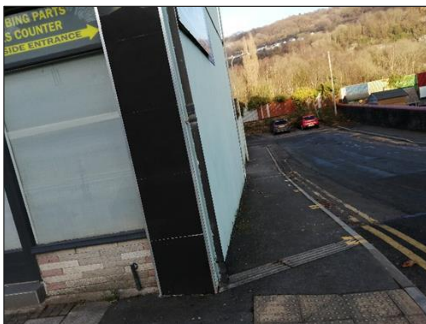
Figure 6: A view of Nile Road from Broadway. (Redstart's Flood Investigation Report)
