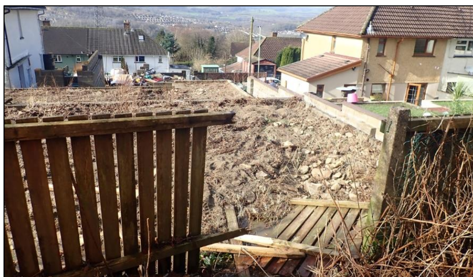
Figure 9: Damages to rear garden of a property at Heol Mynydd following the storm event (captured by FRM officers on 17 th February 2020)
