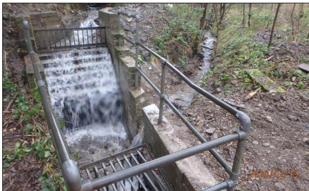
Figure 18: Photo of 'Culvert Inlet 6' captured by RCT's Flood Risk Management team following debris clearance post Storm Dennis (19/02/2020)
