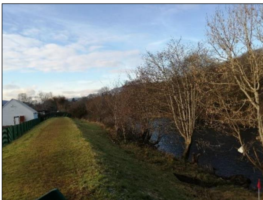
Figure 3: A view of the River Taf and southern riverbank, looking north-east (Redstart's Flood Investigation Report)
